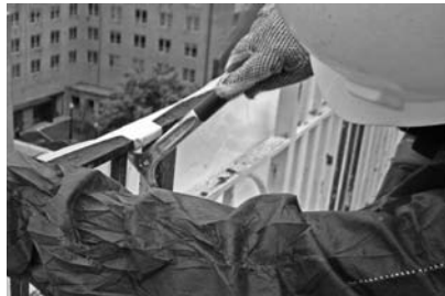
▲ Removal of a failed coating.
