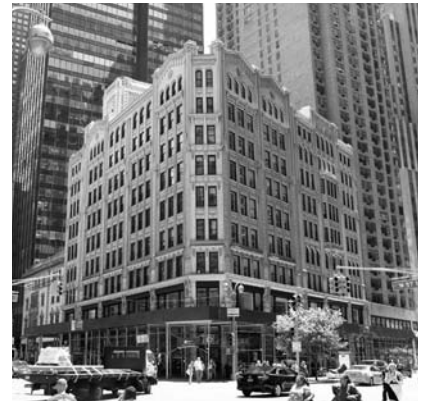
▲ The Argonaut Building, 224 West 57th Street in New York, New York. Terra Cotta Restoration and Coating Replacement.
