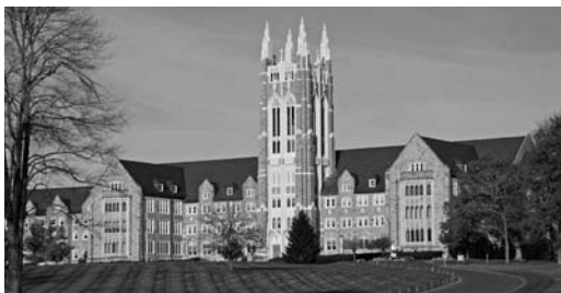
▲ Saint Thomas Seminary in Bloomfield, Connecticut. Bell Tower Facade Rehabilitation with Limestone Coating Replacement.
