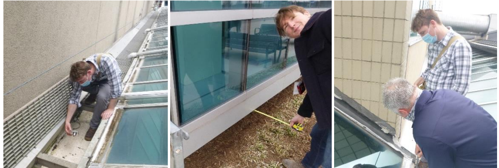
Daniel L. Bishop, AIA on site at roof, curtain wall, and skylight projects in the mid-Atlantic area. Bishop earned a promotion to Senior Architect and celebrates 10 years with Hoffmann Architects.
