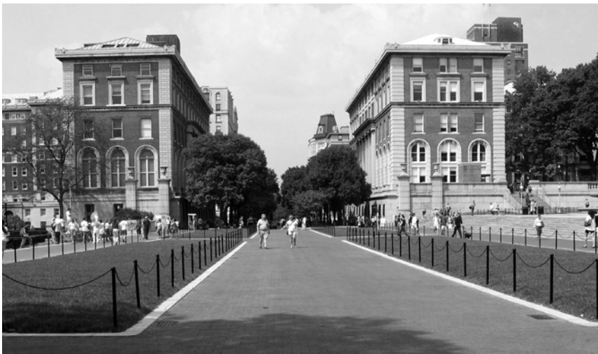
A The reconstructed pedestrian street. The redesigned paving system can withstand frequent, heavy pedestrian traffic, as well as vehicle use, while preserving the aesthetic character of the original plaza.
