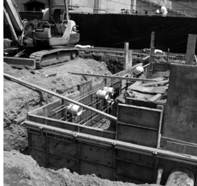
A Construction of concrete retaining walls.
