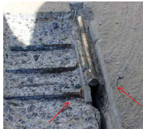
Figure 36 Cracking at concrete and corrosion of rebar due to large weld at stainless steel embedment.
