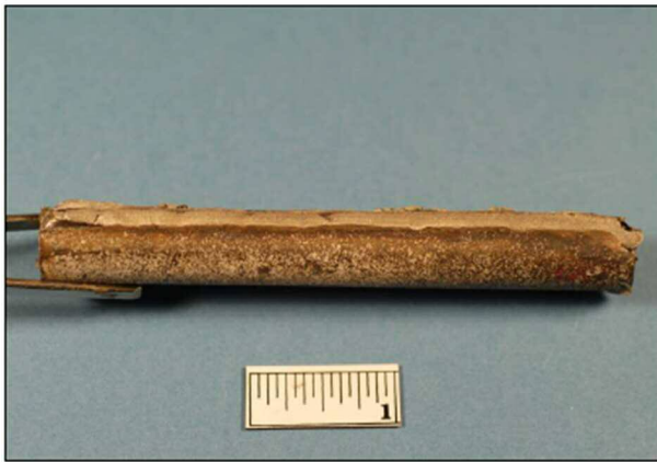
Figure 10A Fatigue failure of a dowel-type connection.
