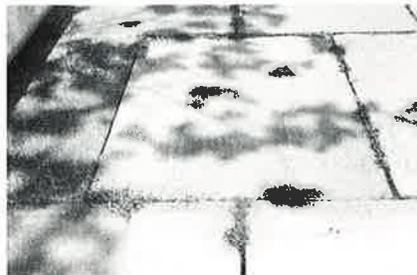
While open joint plazas have many practical and visual advantages, maintenance is important to prevent debris (in this case, pine needles) from clogging the joints and drainage system underneath.
