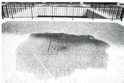
Closed joint plazas are separated into individual watersheds. Increasing the pitch of the surface immediately surrounding the drain can prevent puddles from spreading too far when drains clog, as they often do.
