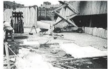
Open joint plaza slabs are relatively easily removed and replaced for inspection, cleaning, and repair. Lack of mortar joints eliminates many maintenance problems common in closed system plazas.
