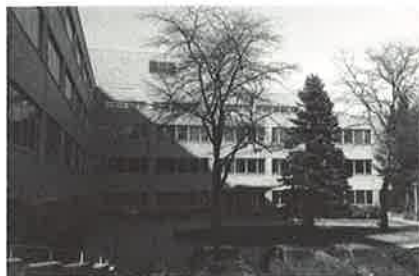
NYNEX Building, White Plains, NY
