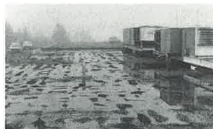
Ponding and Heavy Blistering
