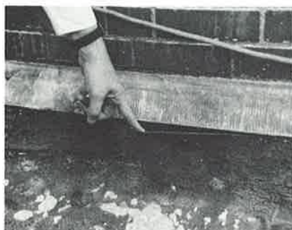
Loose Flashing
