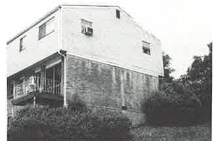
chalking caused white stains on brick
