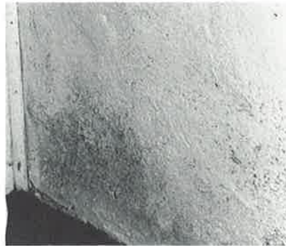
mildew on a painted concrete wall
