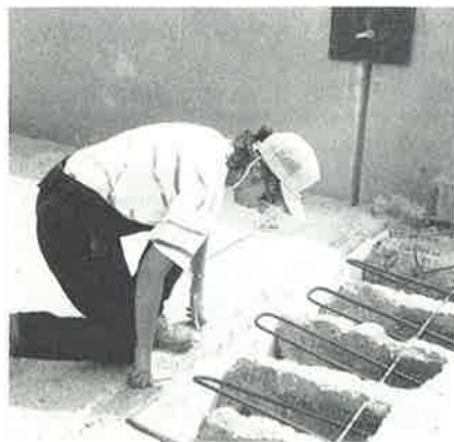
Jane examines repairs to a precast concrete parking garage
