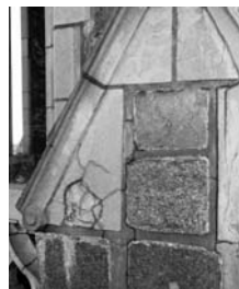
A Before a coating is applied, the substrate must be restored to a smooth, sound condition.
