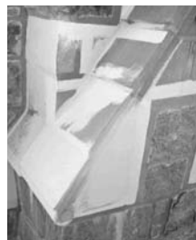
A Before a coating is applied, the substrate must be restored to a smooth, sound condition.
