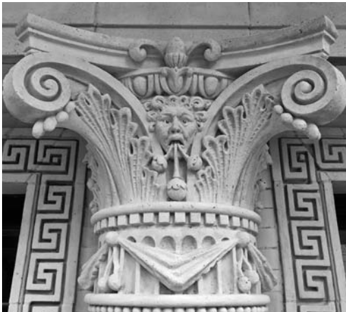
A The coating on this decorative terra cotta element protects the surface from exposure.
