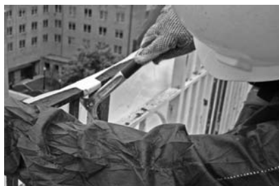
▲ Removal of a failed coating.
