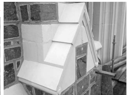
A Before a coating is applied, the substrate must be restored to a smooth, sound condition.
