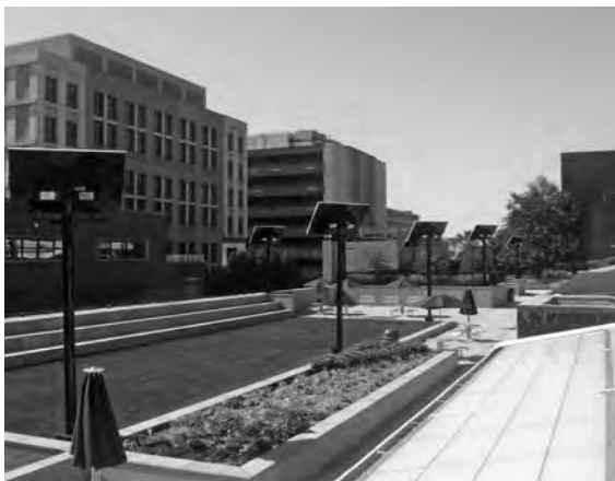
▲ New Jersey City University, Michael B. Gilligan Student Union in Jersey City, New Jersey. Roof Replacement – Intensive Green Roof and MBR System with Reflective Cap Sheet.
