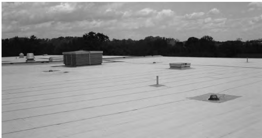
A The white cap sheet on this cold-applied modified bitumen roof assembly reflects solar radiation and disperses heat energy away from the building, keeping the interior cool.
