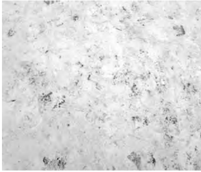
A Dirt and stains from foot traffic can compromise cool roof performance.
