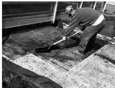
A Remediating a leak on a green roof involves removal of plants and overburden.
