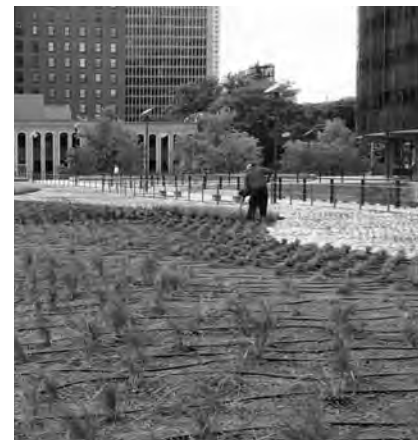
▲ Phoenix Companies Headquarters in Hartford, Connecticut. Plaza as Green Roof – Intensive Roof Garden over Offices and Garage.
