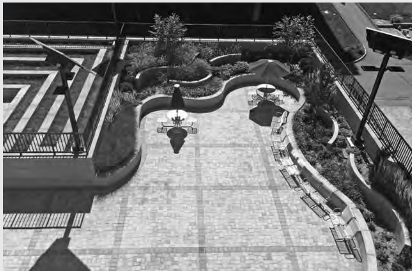
▲ The rehabilitated garden roof terrace at this university student union provides appealing green space for dining, outdoor performances, and other leisure activities.
