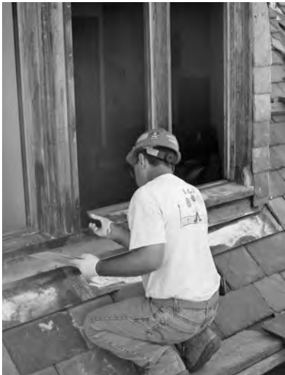
▲ A carpenter restores wood window casing using epoxy repair materials.
