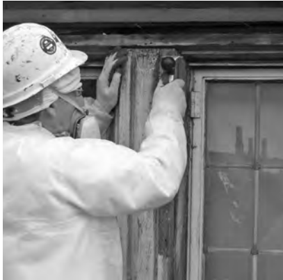
▲ Contractor removing lead-based paint wears personal protective equipment.
