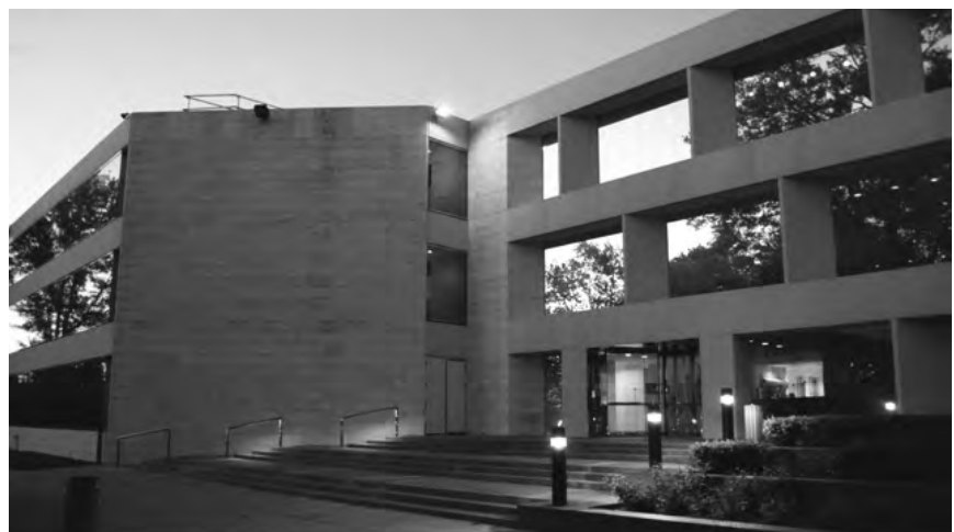
▲ MasterCard Headquarters in Purchase, New York. Plaza and kitchen waterproofing investigations and rehabilitations.
