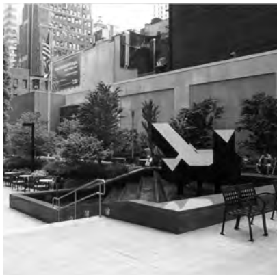
▲ Fountains demand extra attention to waterproofing detail, especially when over occupied space.
