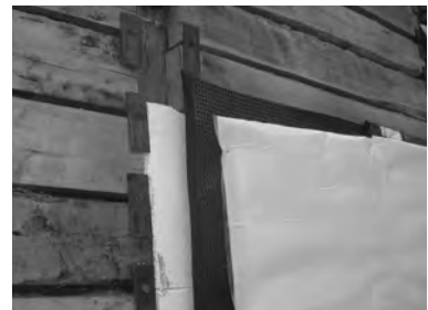
▲ Blind side waterproofing sheet with drainage composite, installed prior to concrete.
