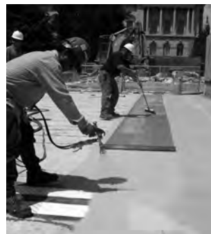
▲ Application of deck waterproofing with reinforcing fabric.
