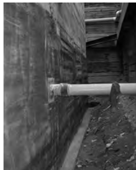
▲ Spray-applied liquid waterproofing.
