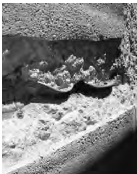
▲ Bent water stop in vault wall.
