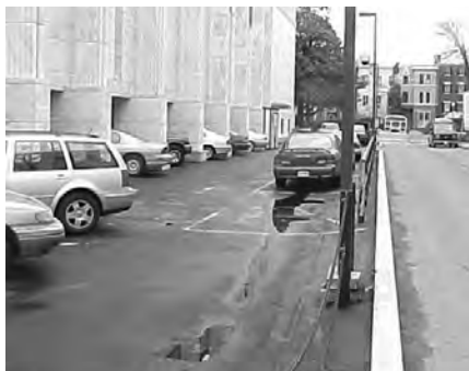
▲ Below-grade vault is under parking deck.
