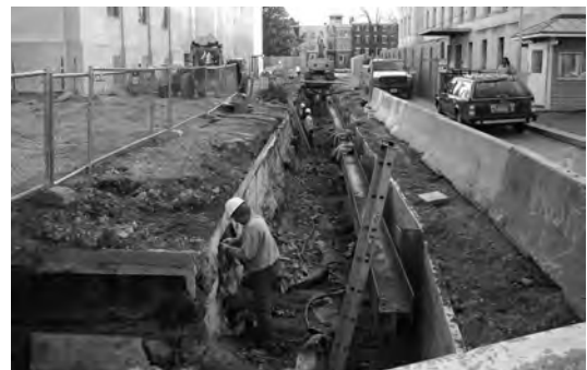
▲ Excavation to expose vault and deficient waterproofing.
