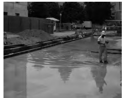
▲ Flood test of waterproofing on rehabilitated deck.
