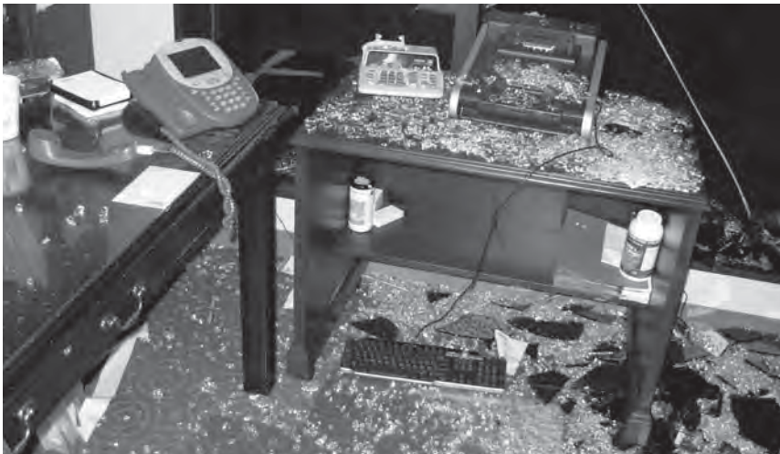
▲ Even a small breach in the building envelope can lead to serious devastation as tremendous wind pressures build inside the structure.
