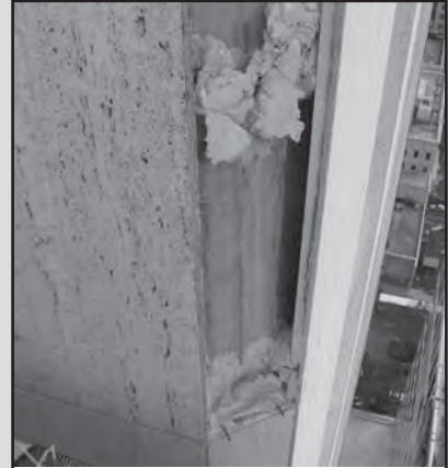
A Insufficient load capacity compromised the wind resistance of these panels, which otherwise might have remained intact.
