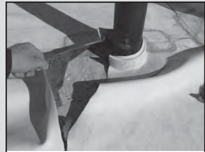
▲ Poor anchorage and weak membrane adhesion were signs that this roof failure could have been avoided.
