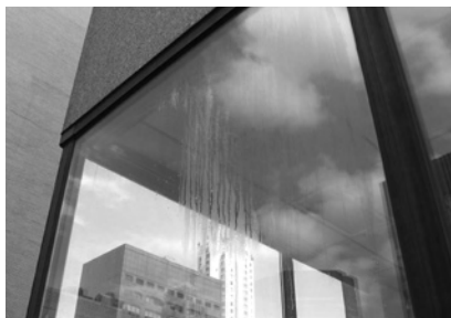
▲ Condensation doesn't just cloud the view, it points to poor thermal performance.
