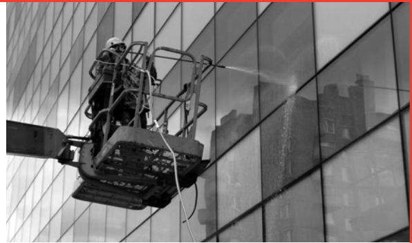
▲ Commissioning often includes performance testing, such as water intrusion tests, to see that assemblies react as designed.
