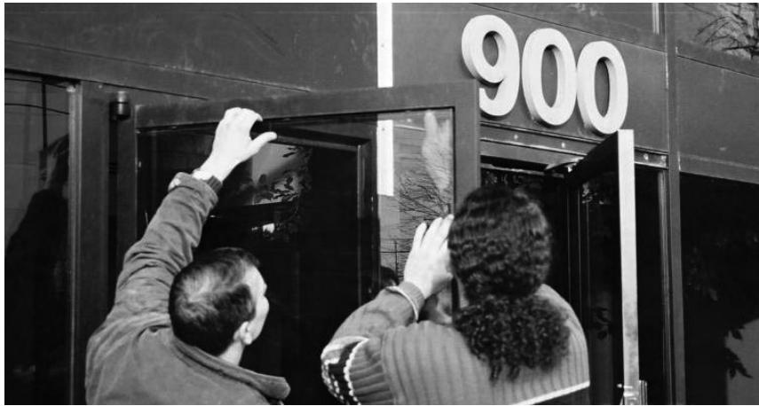
A Poorly performing doors make HVAC systems work overtime to stabilize temperature.
