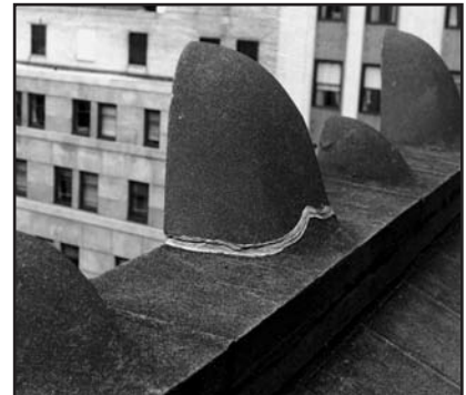
▲ Inappropriate “band-aid” repairs are not only unsightly, they create additional impact on the environment when they fail or, worse, damage surrounding building elements, which in turn require repair.
