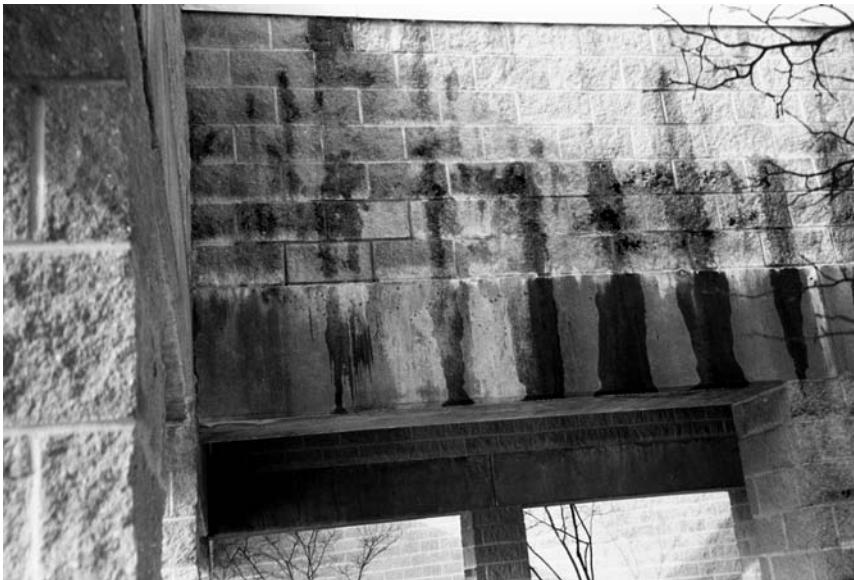
▲ Failure to properly detail and build this concrete block wall left it open to water entry, which led to toxic mold growth. Exterior wythes must be demolished and rebuilt, wasting materials and energy.
