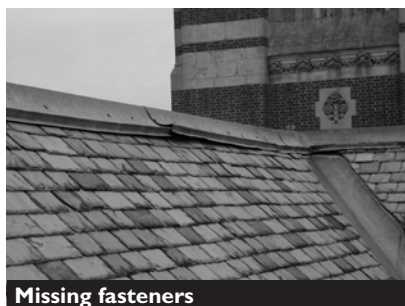
Missing fasteners
