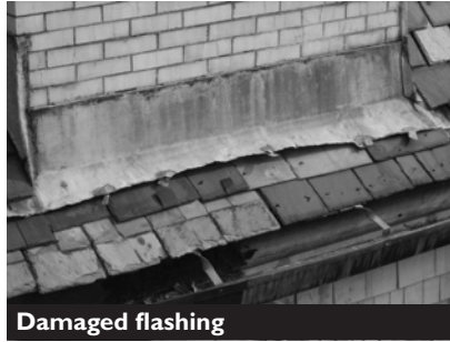
Damaged flashing
