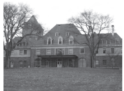
▲ Fairfield University, McAuliffe Hall (pictured), and Bellarmine Hall in Fairfield, Connecticut. Slate Roof and Building Envelope Rehabilitation
