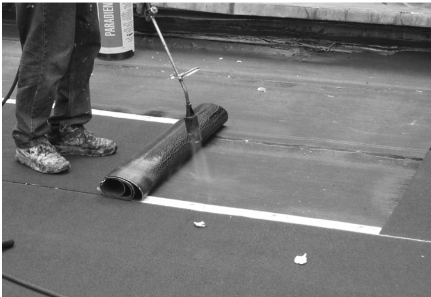
■ Torch-applied ( left ) and cold-applied MBRs (see photo on page 4 ) provide the resilience and durability of traditional built-up systems, without the need of lifting or pumping 400°F molten asphalt onto the roof ( above ).
