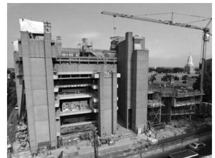
▲ Art and Architecture Building at Yale University in New Haven, CT. Building Envelope Rehabilitation, including Roof Replacement.
