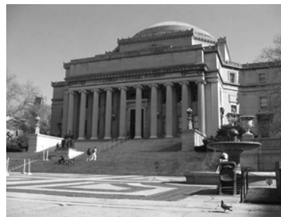
▲ Low Memorial Library at Columbia University in New York, NY. Roof Replacement.
