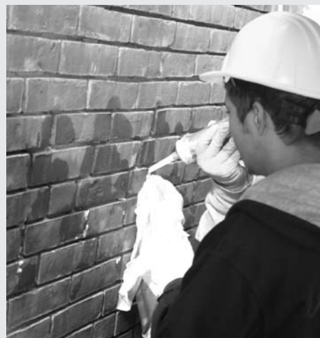
▲ Workers inject mortar into the thin joints of a historic building.
