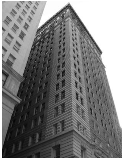
▲ 25 Broad Street (1902) in New York, NY. Exterior Rehabilitation.
