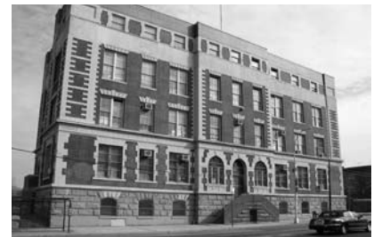
▲ Public School 36 (ca. 1901) in Bronx, NY. Masonry Façade Rehabilitation and Window Replacement.
