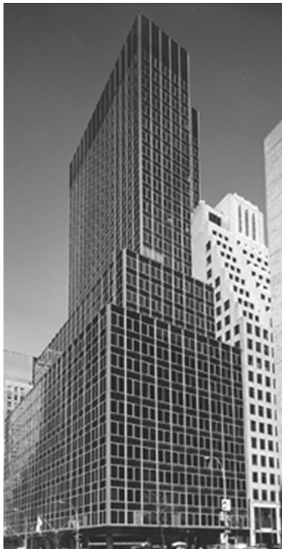
A Curtain walls may be rehabilitated for aesthetic reasons or to improve energy efficiency, in addition to the need to resolve deterioration associated with weathering, age and materials or installation failures.
