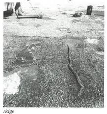
*SLIPPAGE* – If the slope is too great for the type of bitumen used, or poor installation allows the felts to slide, repair by mechanically fastening the membranes through the insulation to the decking. The fastener disk should be set in roofing cement then flashed in with two layers of fabric and roofing cement following the procedures described under "Blisters." Each row of fasteners should run parallel to the slope.
