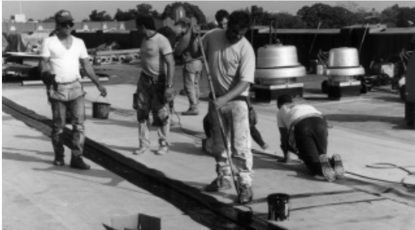
Adhesive is applied to a lap splice in an EPDM membrane.
