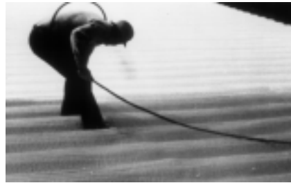
A worker applies silicone coating to a urethane foam roofing system.
