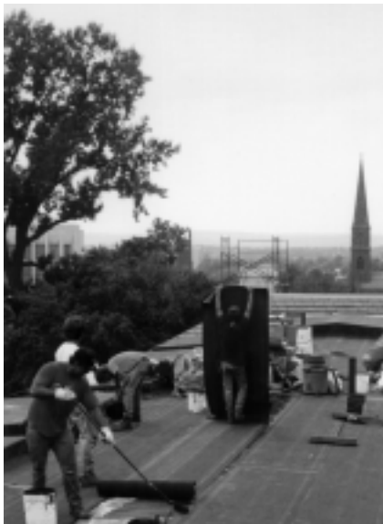
Workers install a cold-applied modified bitumen roof (MBR).
