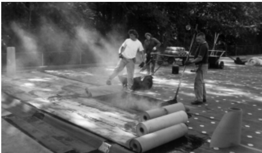
Workers apply built-up roofing (BUR) over fastened insulation.
