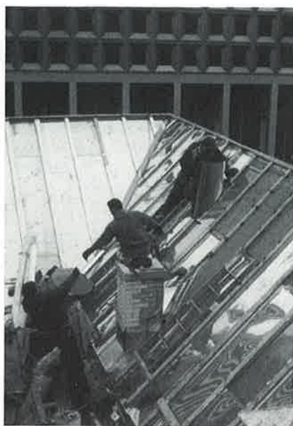
Installation of a batten seam copper roof on a New York City high-rise office building.
