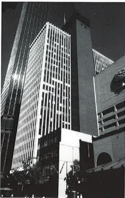
Midwest Plaza Garage in Minneapolis, Minnesota
