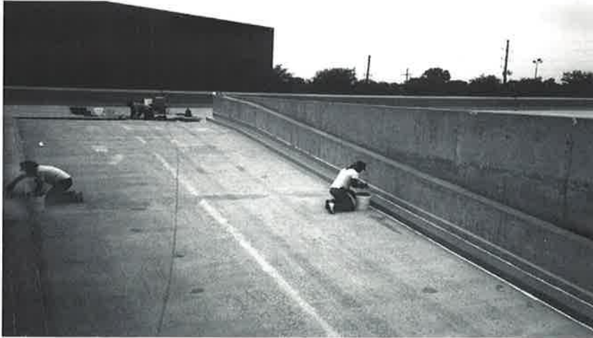
Application of urethane detail coat prior to base coat installation.
