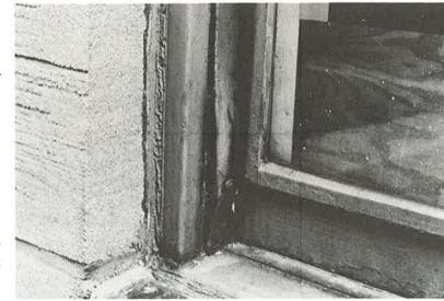
Severely corroded window jamb
