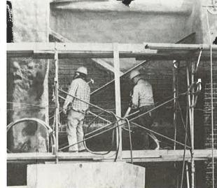
application of shotcrete over wire mesh reinforcing.
