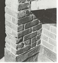
ing which allows more water to enter the wall and corrode the steel spandrel beams. The rust expands, causing further cracking.
