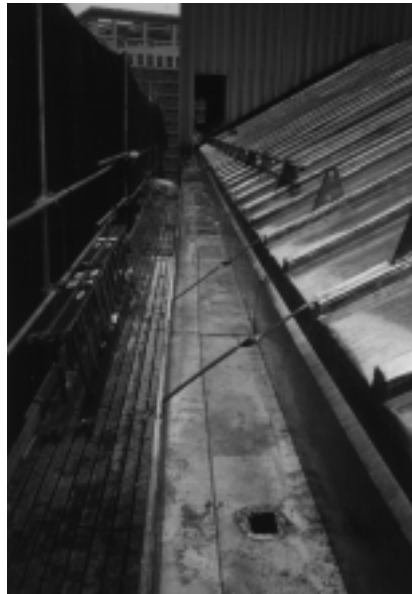
A batten seam roof edge with hung gutter and snow guards.
