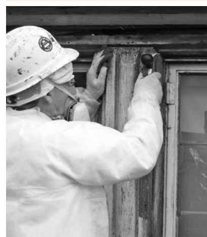
A Hazardous materials abatement requires critical barriers and appropriate phasing.
