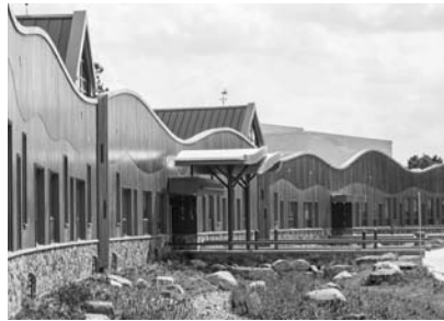
▲ Sandy Hook Elementary School , Newtown, Connecticut, Exterior Envelope Consultation.
