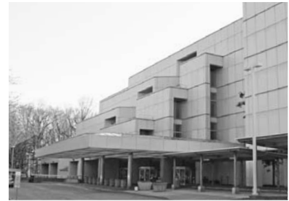
▲ Social Security Administration, National Computer Center , Woodland, Maryland, Facade Repairs.
