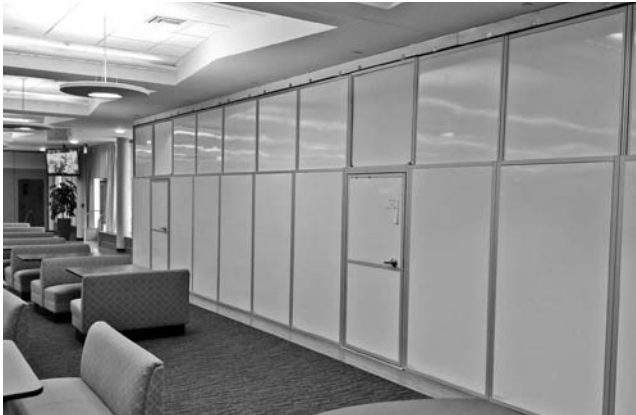
A Temporary interior partitions provide both a physical and a visual barrier, maintaining building operation until construction is completed.
