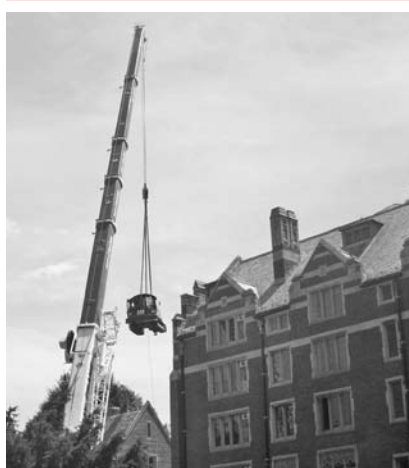
A Where the job site is difficult to access, equipment may need to be lifted by crane.
