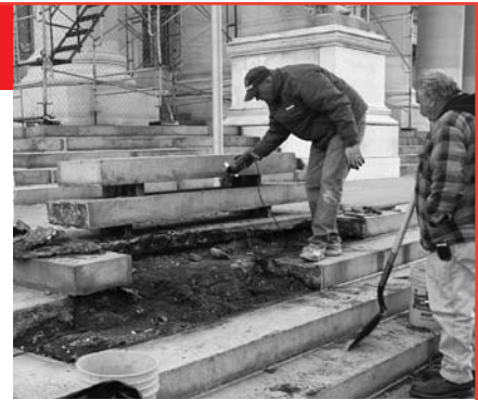
▲ At this historic courthouse, maintaining security during restoration was a key concern.
