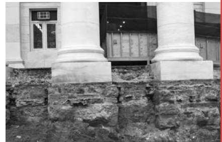
▲ Temporary ramps provided controlled access while the stairs were reconstructed.
