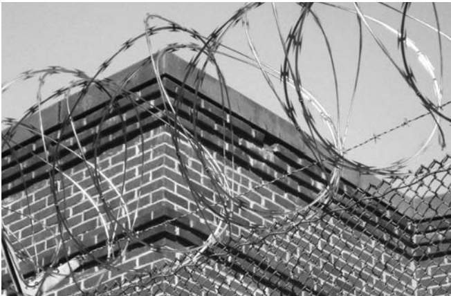
▲ With the right planning, building envelope deterioration can be addressed at any facility, even those with the highest level of security.
