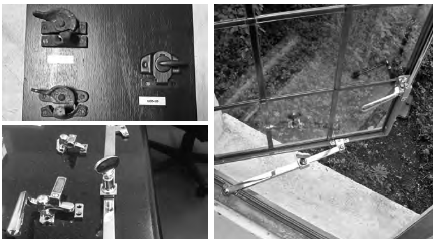
▲ Samples of original hardware (top left) facilitate restoration and, where necessary, replacement. Existing historic hardware may be removed and restored (bottom left), then re-installed (right).
