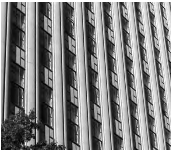
▲ Meeting performance demands while preserving building character presents challenges for historic window projects.
