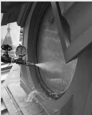
▲ Water test of newly installed window.
