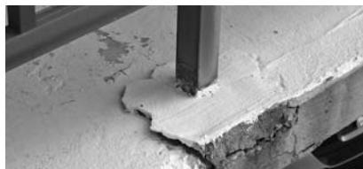
▲ Railing corrosion causing cracks and spalls at post-slab interfaces (left) and exterior walls (right).
