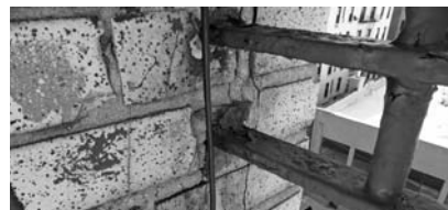
▲ Railing corrosion causing cracks and spalls at post-slab interfaces (left) and exterior walls (right).
