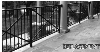
▲ New railings maintain character of originals, but meet code requirements.
