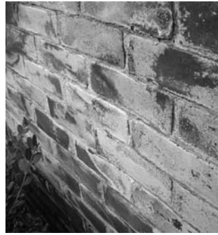
▲ Efflorescence.
