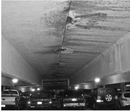
▲ Figures 4a (left) and 4b (right): Corrosion concentrated at flange connections in this precast concrete garage due to inappropriate materials, weld defects, and sealant joint failure.
