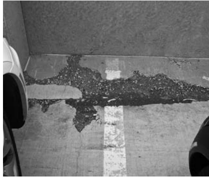
▲ Figures 5a (left) and 5b (right): Insufficient air entrainment of this concrete surface left freezing moisture no room to expand, leading to severe disintegration.
