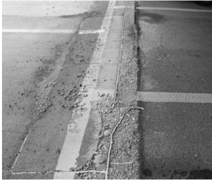
▲ Figures 5a (left) and 5b (right): Insufficient air entrainment of this concrete surface left freezing moisture no room to expand, leading to severe disintegration.
