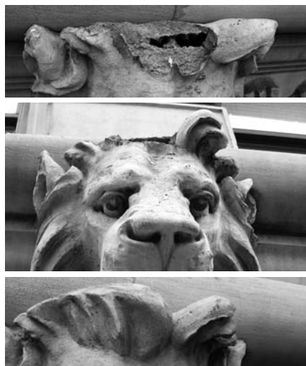
▲ Restoration of spalled terra cotta decorative element.
