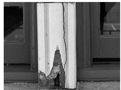
A Crack and spall caused by corroded steel.
