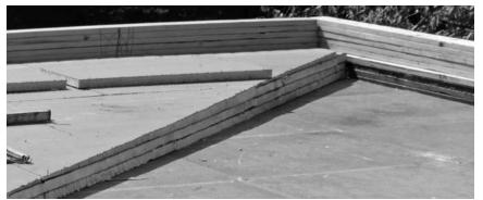
A When adding insulation to the roof, consider the impact on edges, terminations, and transitions, which may need to be adjusted to accomodate the additional depth.
