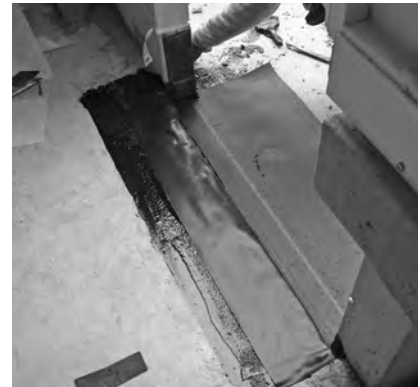
Waterproofing installation review: As potential sources of water infiltration, thresholds demand attention to detail. Here, asphalt and roofing felt ( left ) are applied under the flashing membrane ( center ) to create a positive lap, then the roofing base membrane is embedded into the asphalt ( right ).
