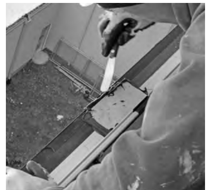
Curtain wall installation review: Creating a water-tight intersection is a multi-step process, beginning with application of sealant at the glazing pocket ( left ), then placement of metal covering over the gap ( center ), followed by appropriate tooling of sealant at the horizontal weather seal ( right ).
