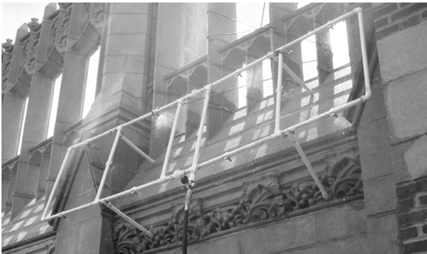
▲ As part of a defect survey, spray rack water tests quantify the extent and location of water penetration.
