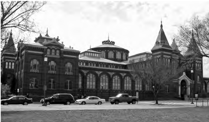
▲ Arts and Industries Building at the Smithsonian Institution in Washington, District of Columbia. On-Site and Off-Site Window Assembly Water Testing.
