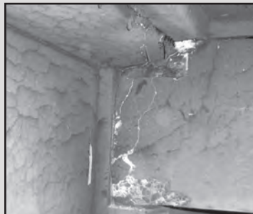
A Sharp edges and color differences were clues that these cracks hadn't been there before the fire.
