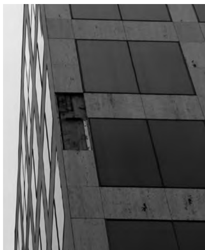
A Insufficient anchorage allowed this stone panel to blow off in a hurricane.
