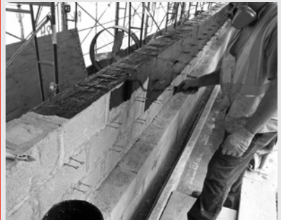
▲ A liquid-applied air barrier provides a continuous layer of moisture protection.
