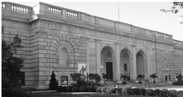
▲ Smithsonian Institution, Freer Gallery of Art, Washington, DC, Mortar and Parapet Leak Investigation.
