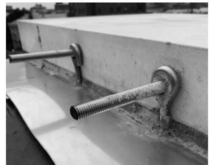
▲ Stainless steel anchors secure coping stones against displacement.
