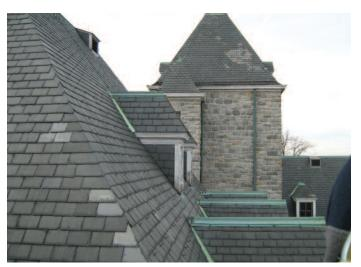
Failure to match the color, profile, and texture of existing slates when selecting replacements can lead to an unattractive patchwork appearance.
