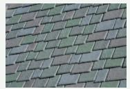
Example of synthetic slate roofing shingles.
